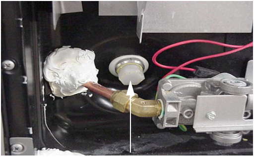
Water Heater Drain Plug (Remove with socket)
