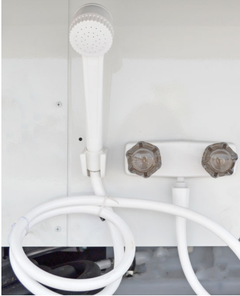
Exterior Shower/Wash Station -Typical View
