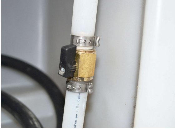
Water Tank Drain Valve -Typical installation shown
